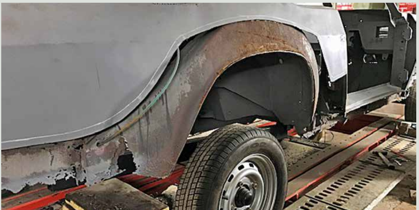
Rear wheel arch stripped and being prepared for welding new arch
