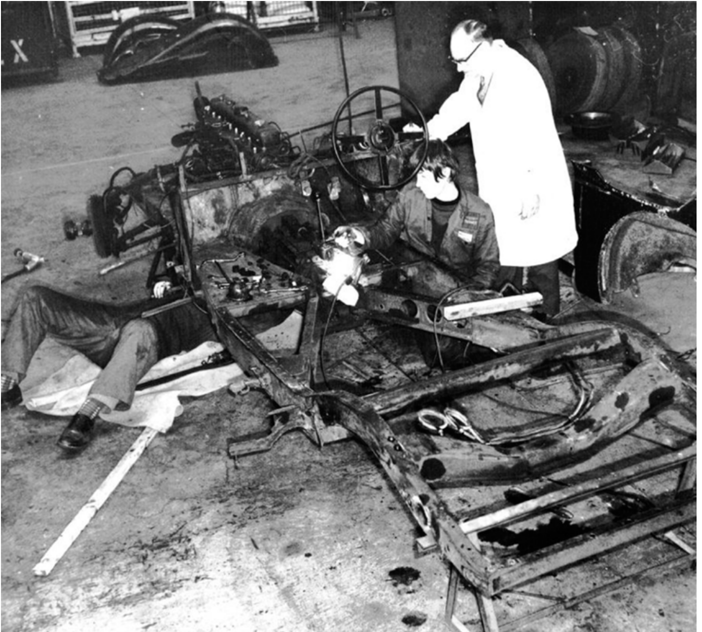
H5 with the body tub, floors, panels and running gear removed
